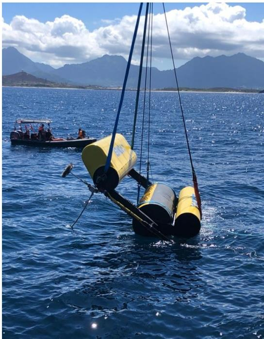
3. Deployment of the Ocean Energy (Ireland) OE35 WEC at the 60m berth. This device has been in Hawai‘i since December 2019, and underwent drydock repairs in August/September 2022, after extensive delays. A new generator was installed in April/May 2024, and it was deployed to WETS in July. However, it is not yet operational, as weather and logistics have not yet supported the operation to connect its umbilical cable to the WETS shore cable. It is hoped this will be achieved soon.
