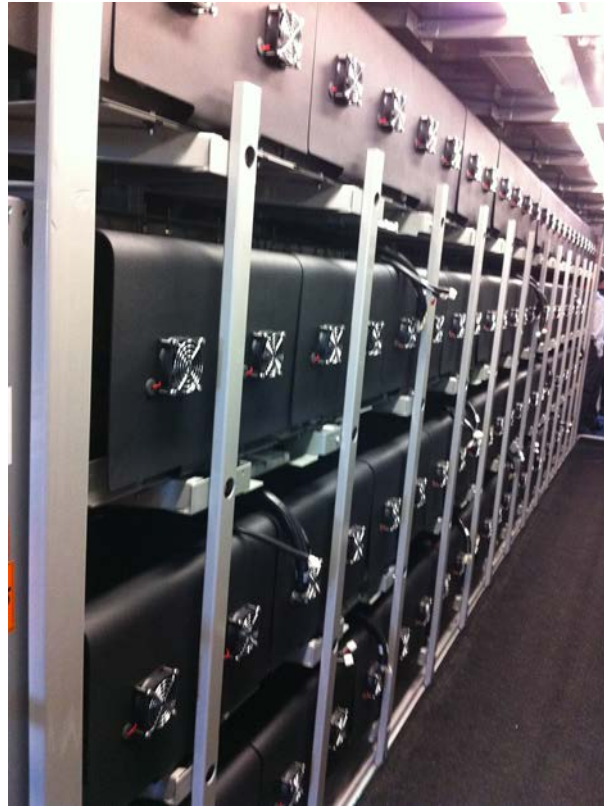
Altairnano (ALTI) 2 MW/333kWhr Battery Energy Storage System (BESS)
