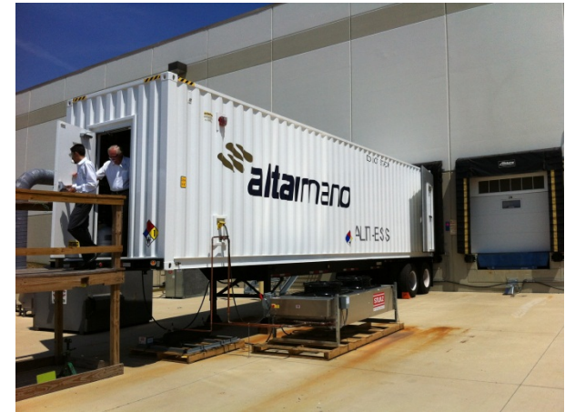
Altairnano (ALTI) 2 MW/333kWhr Battery Energy Storage System (BESS)
