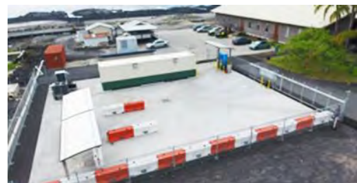
Figure 3. HNEI Hydrogen Station.
