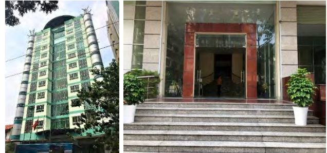
Figure 1. HCM-USTA Building, Ho Chi Minh City.
