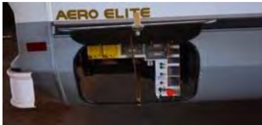
Figure 9. Bus Export Power Unit.
