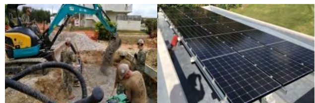
Figure 3. Project construction and new PV system.
