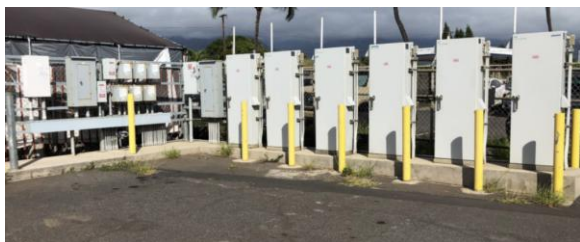
Figure 1. Sunverge SIS BESS + PV units on Maui.
