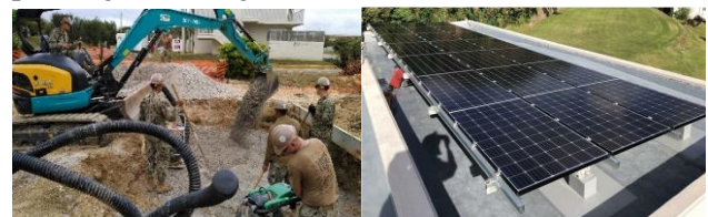
Figure 4. Project construction by Navy Seabees and new PV system.
