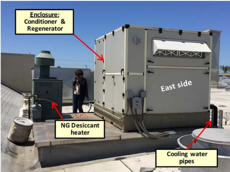
Figure 7.4.5: System housing (enclosure conditioners & regenerator)
