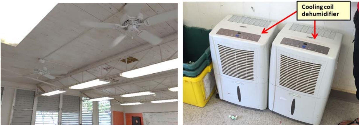
Figure 7.5.6: Mold growth in a space that was considered the most affected by mold, shown are the two portable dehumidifier that were used to lower the humidity level.
