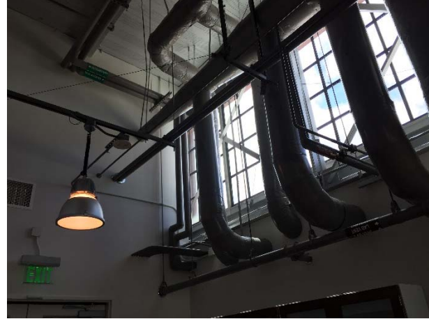
Internal ventilation and cold-water pipes
