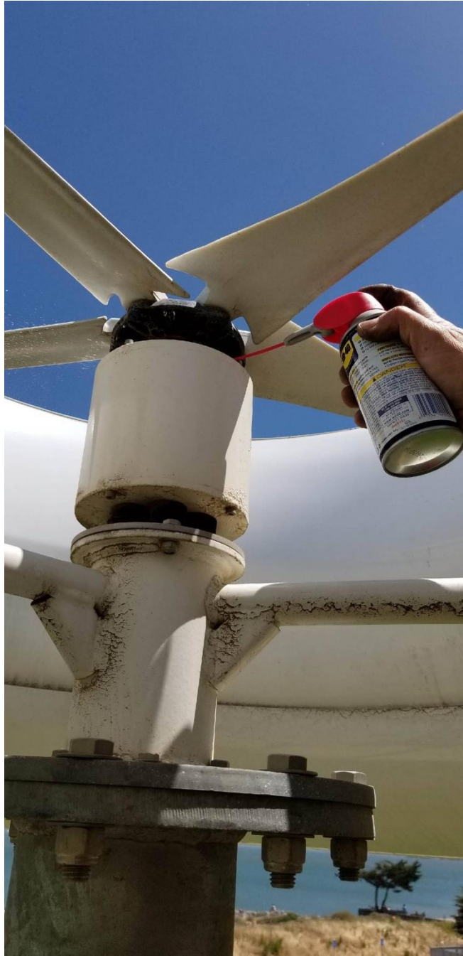
Figure 8. WD40 in moving parts to reduce risk of future seizing
