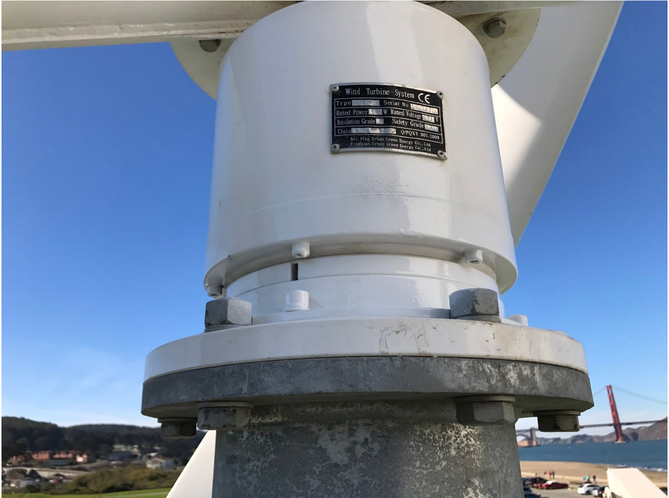
Rustoleum flat protective enamel was applie to rusted areas on turbine.
