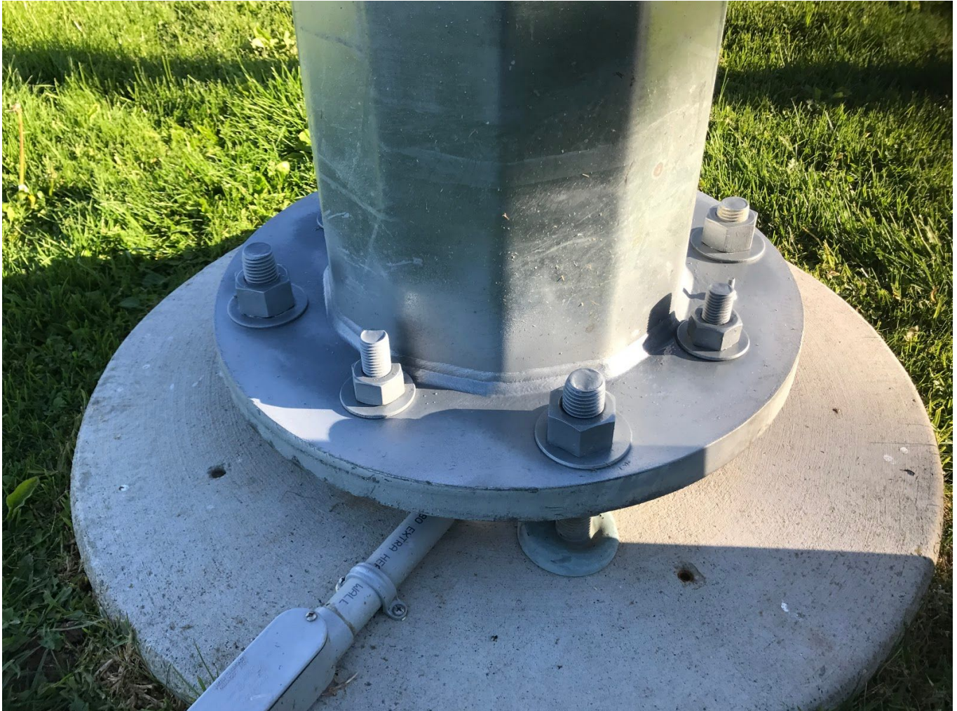
Rust occurred on hardware on bottom of posts. Cold galvanizing compound was applied
