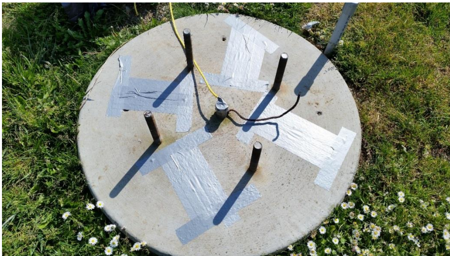
Figure 8: Foundation top prepared for drilling.
