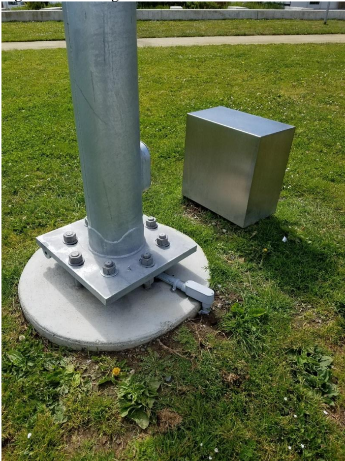
Figure 28: Completed turbine base installation with disconnect housing.
