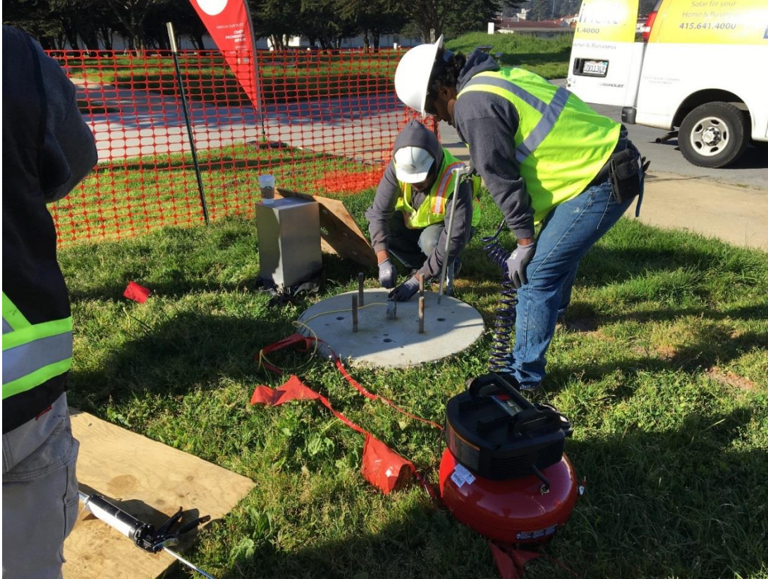
Figure 8: Drilling holes in the existing Windspire foundations.
