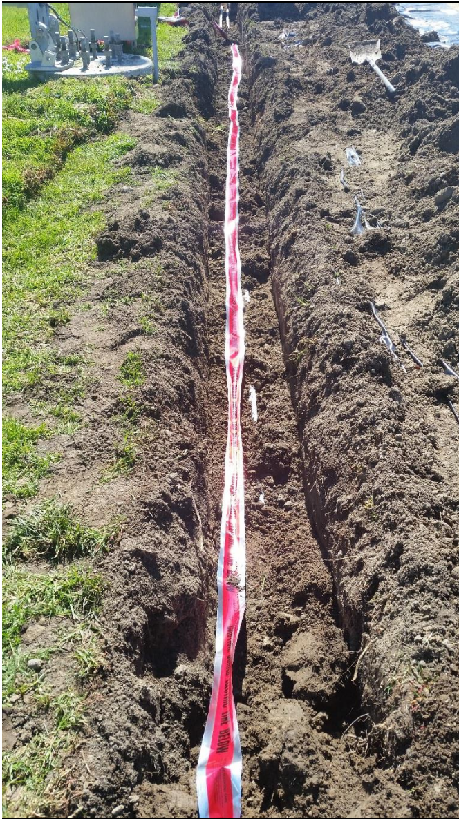
Figure 22: Detection tape.
