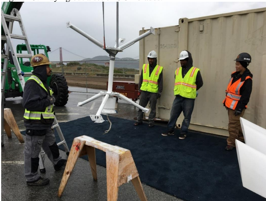
Figure 14: Preparing UGE generator/shaft for blade installation.
