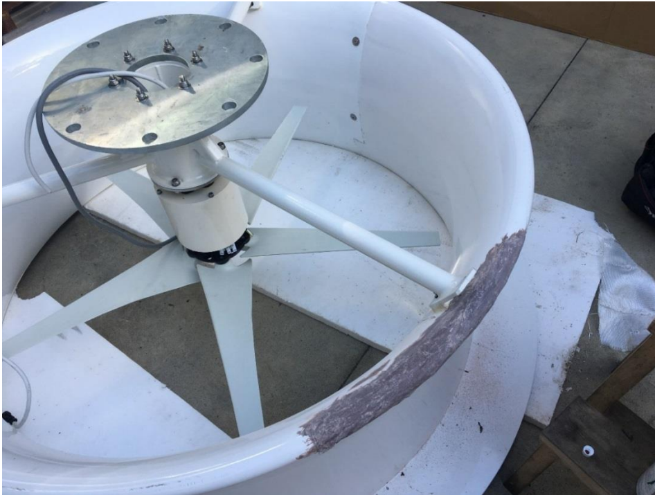
Figure 1: Minor shipping damage was observed on one of the Omniflow cowlings when it was unpacked. Here the unit is shown undergoing repairs with an epoxy compound.
