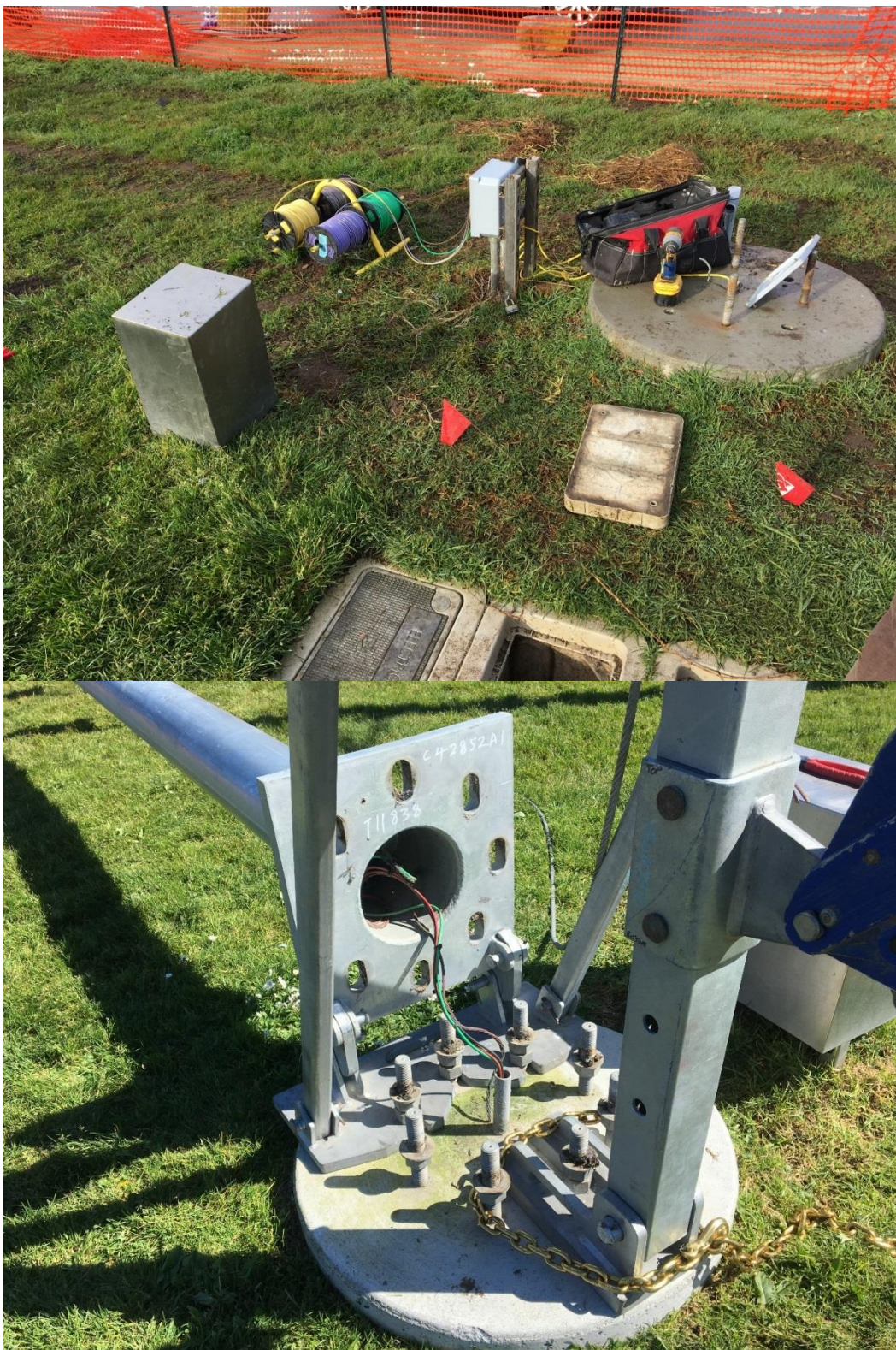
Figures 25 & 26: Wiring a turbine and disconnect switch.
