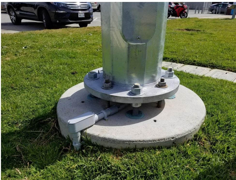
Figure 12: UGE tower installed and bolted in.
