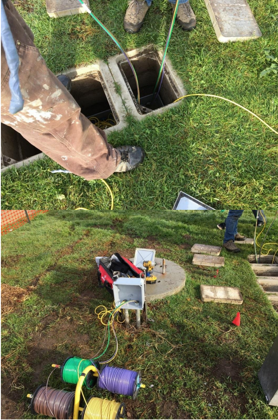
Figures 23 & 24: Pulling conductors.
