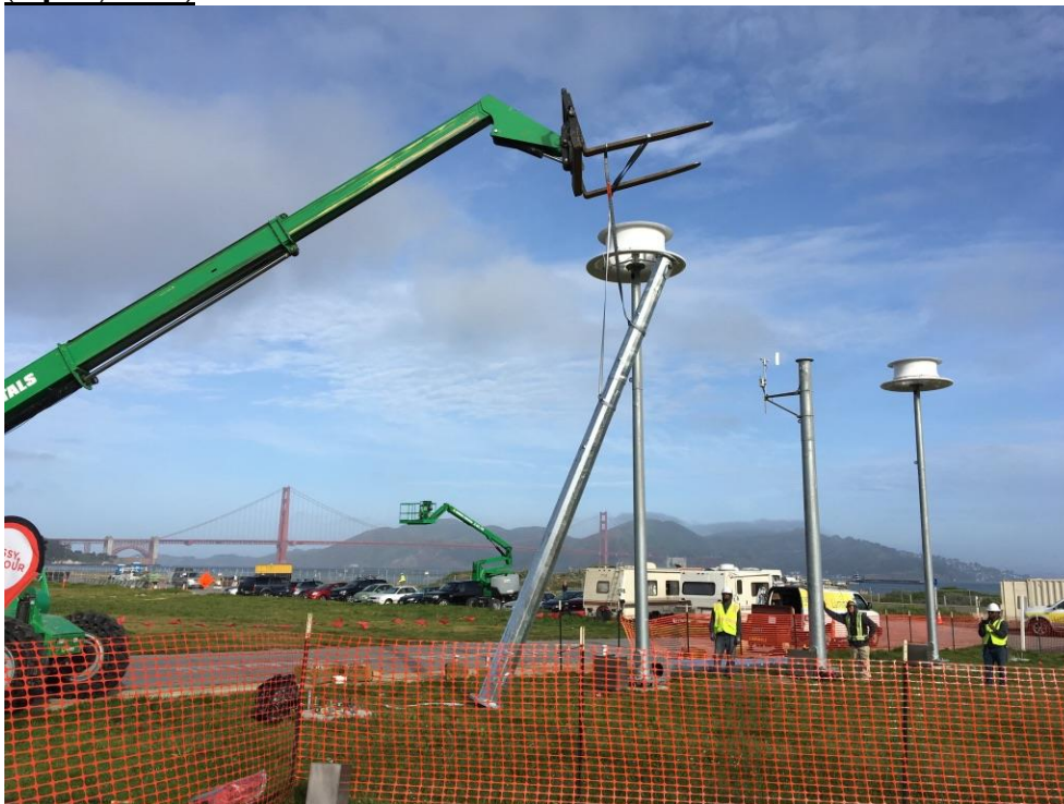
Figure 11: Setting UGE South tower on retrofitted foundation.
