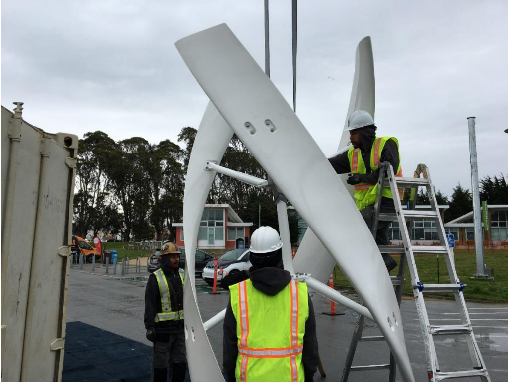
Figure 15: UGE blade assembly.
