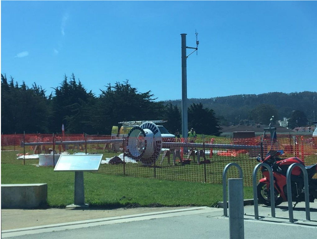
Figure 3: North Omniflow unit assembled on tower and ready to raise into place.
