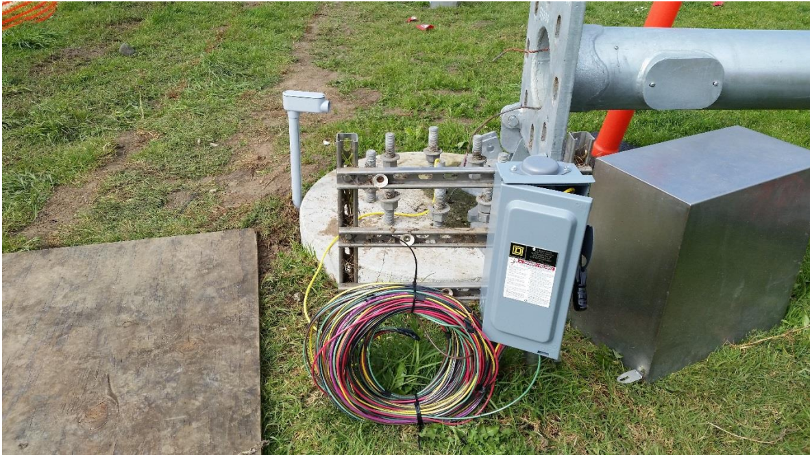
Figure 27: Wiring a turbine and disconnect switch.
