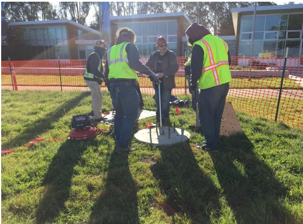
Figure 9: Cleaning and prepping new anchor bolt holes.
