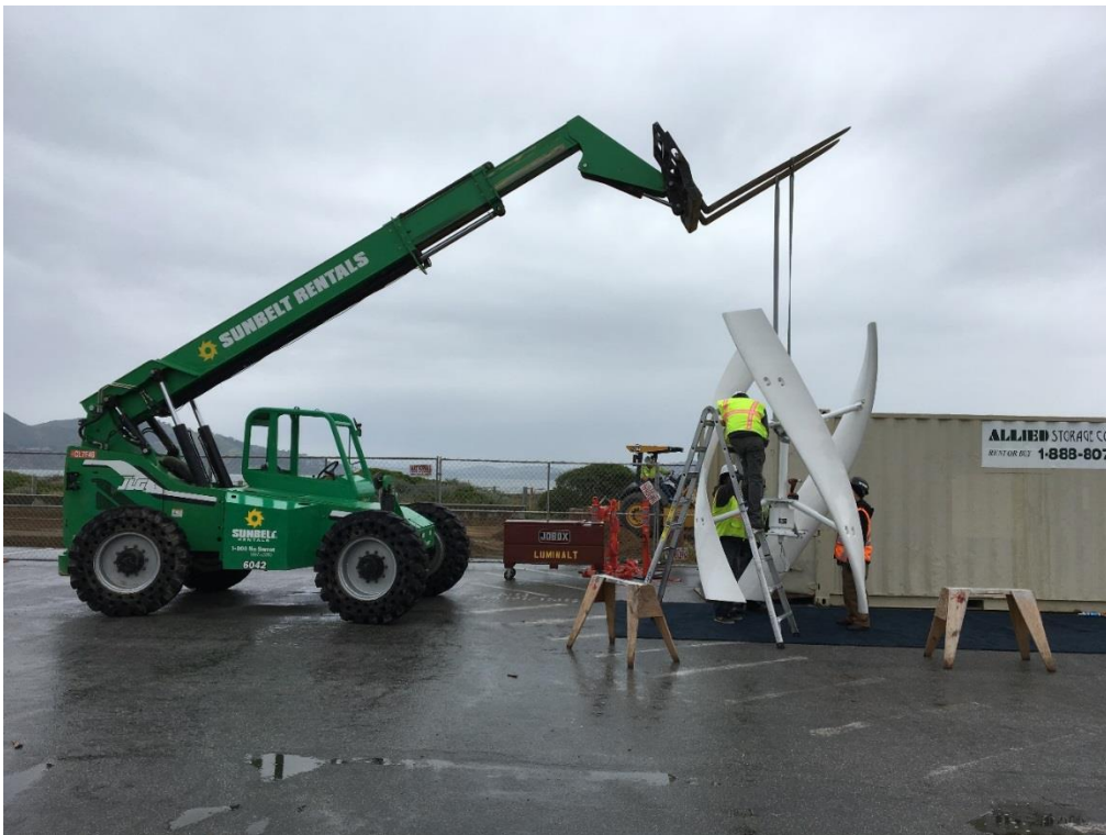
Figure16: UGE turbine head ready for installation on tower.
