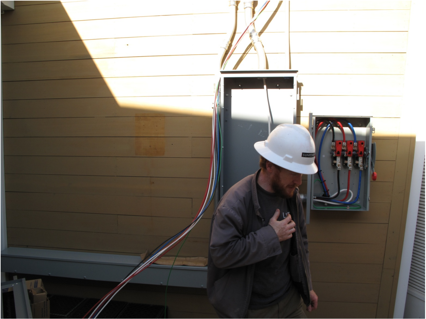
Tie in to Renewable Energy sub-panel in progress
