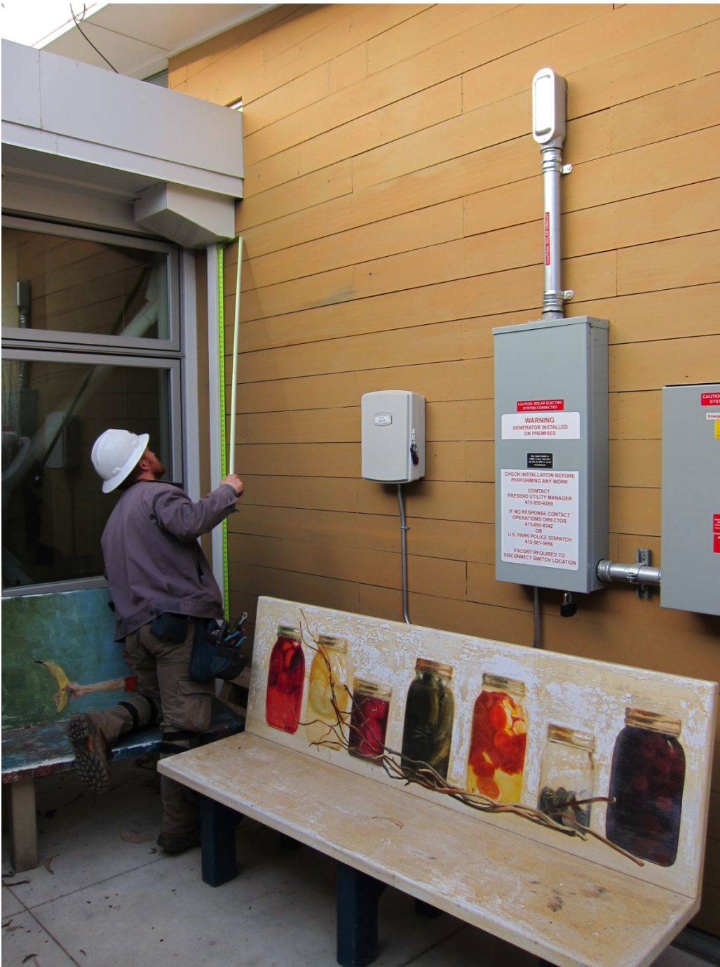
Laying out Inverters and Rectifiers
