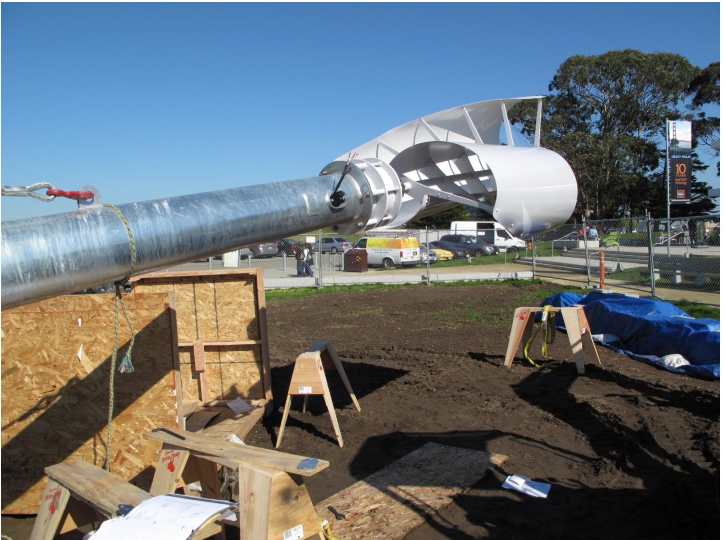
Tangerie unit mounted to tower
