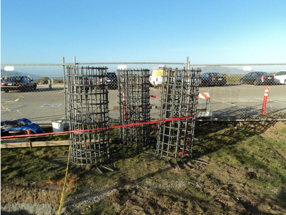
Tower Cage Rebar Prepared
