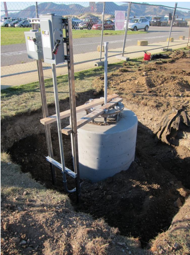
Completed Footing with Disconnect/Brake Switches
