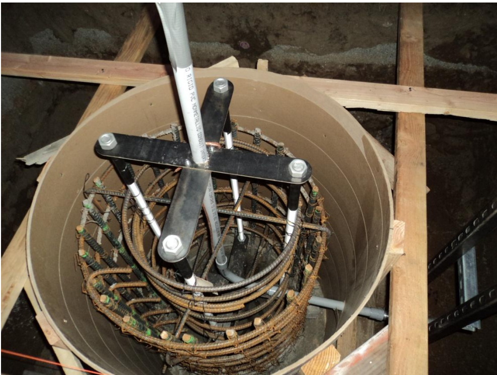
Windspire Footing Encased in Sonotube
