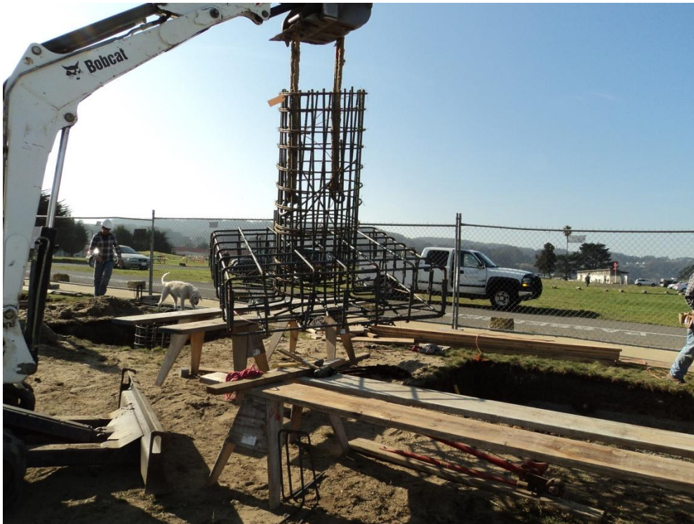
Rebar Placement
