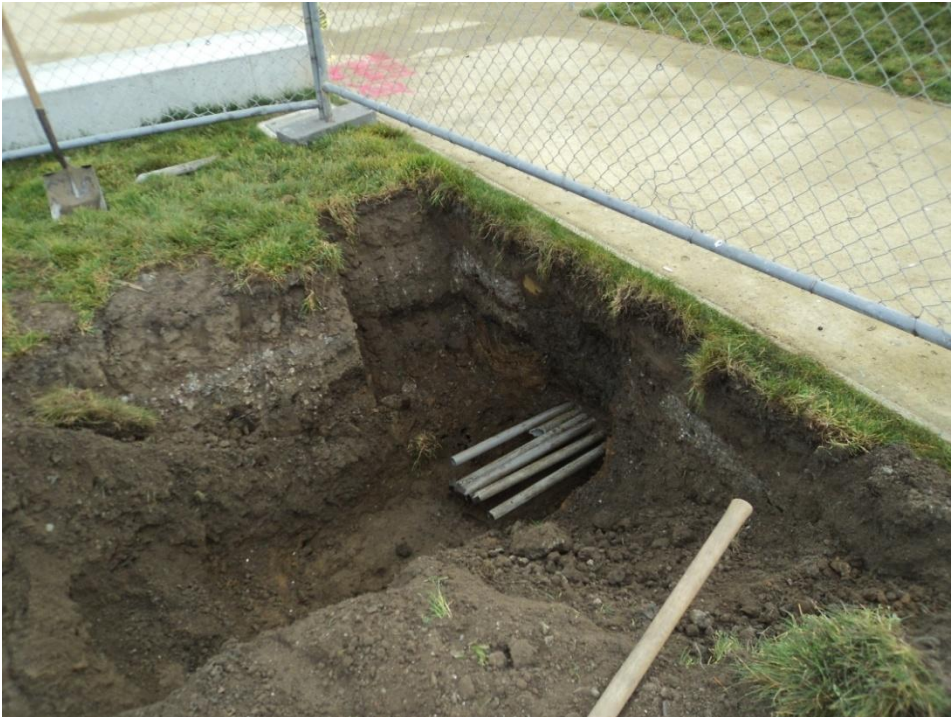
Pre-Installed Conduit Run to Building
