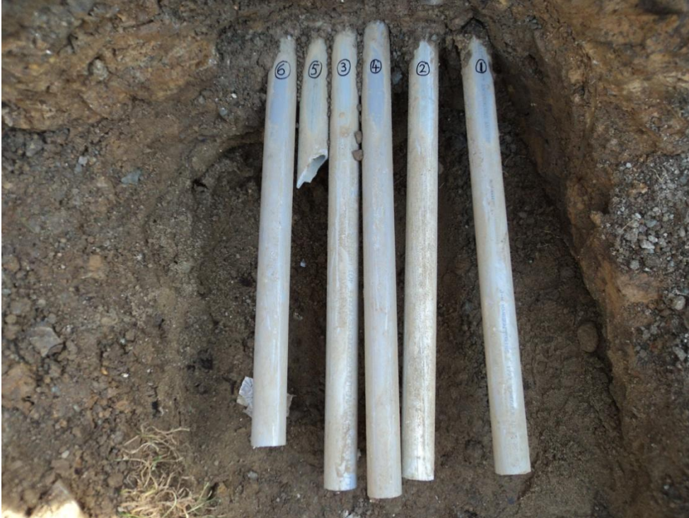
Pre-Installed Electrical Conduit Run to Building
