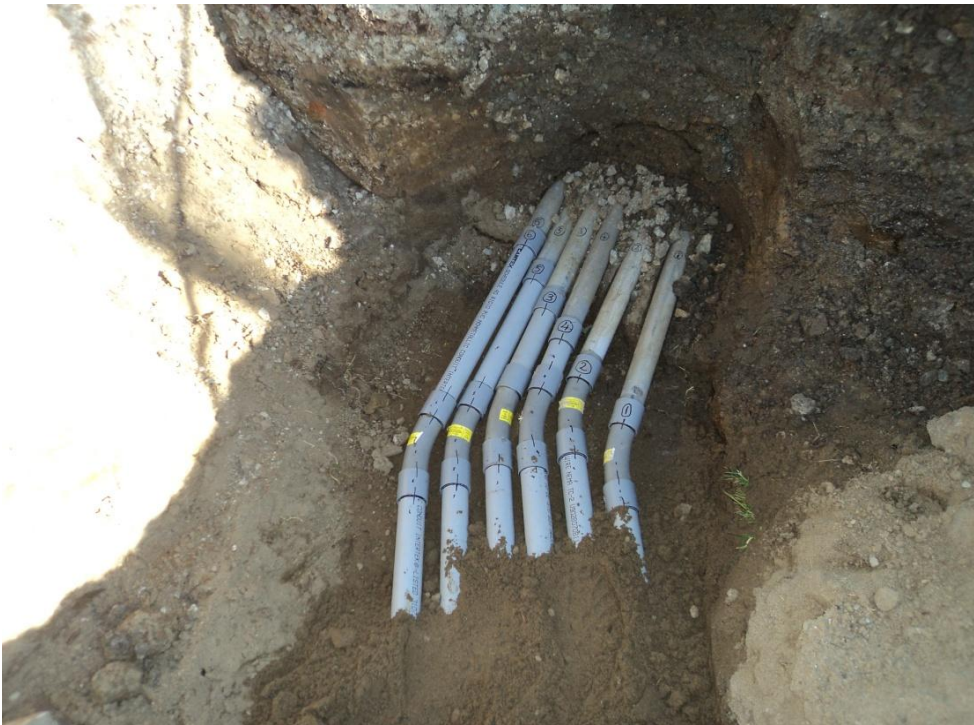
Connection: Facility to Turbine Electrical Conduit
