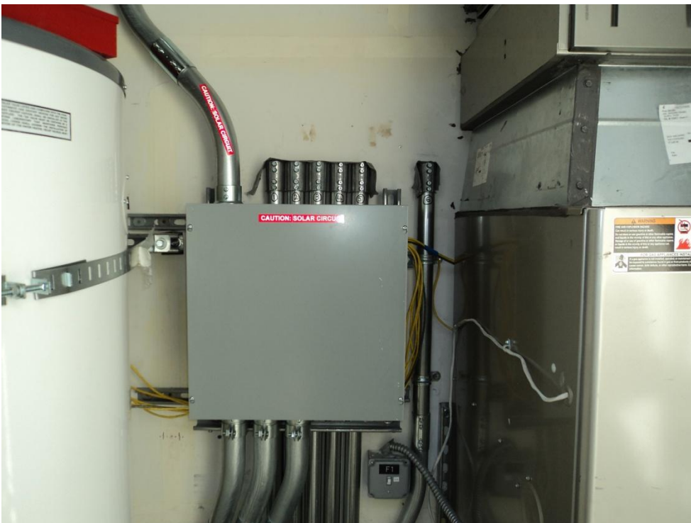
Electrical Conduit At Mechanical Closet
