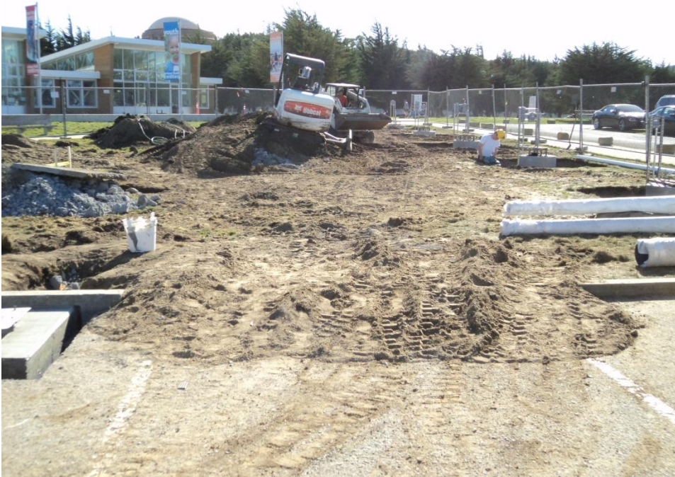
Backfill in Progress
