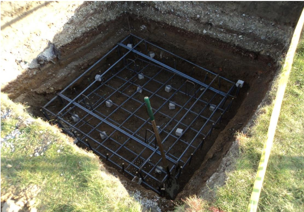
Rebar Installation Start
