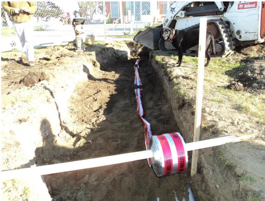
Detection Tape at Conduit Trench: Ready for Backfill
