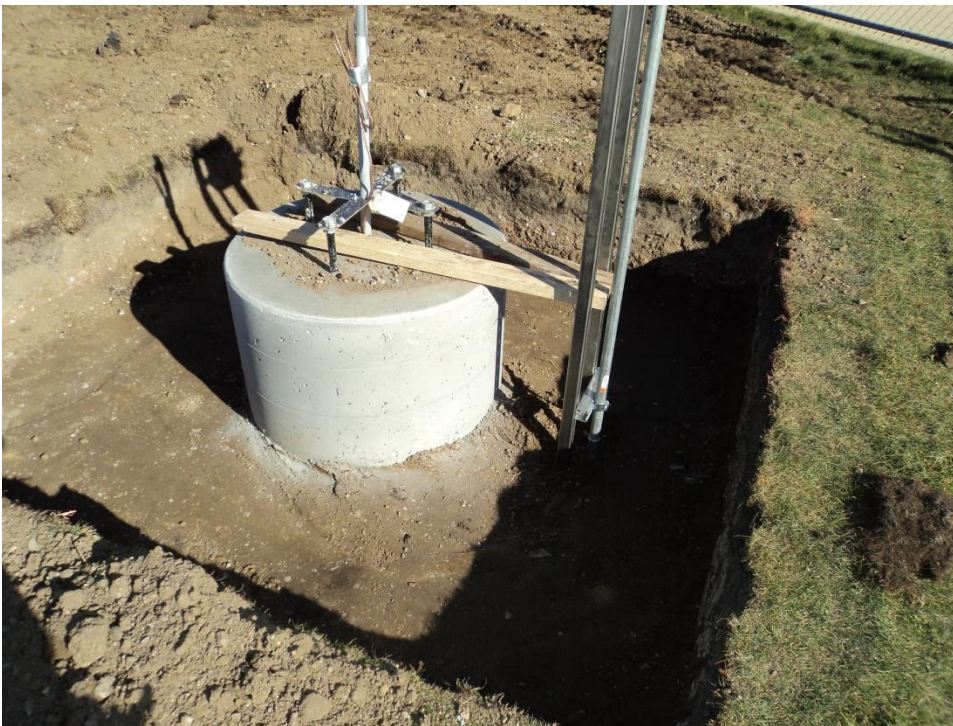
Backfill at Footings, by 6" Lift
