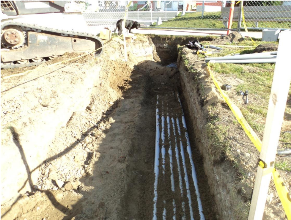
Main Conduit Distribution to Turbines
