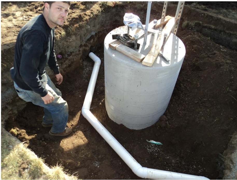
Typical Conduit Distribution to Turbines
