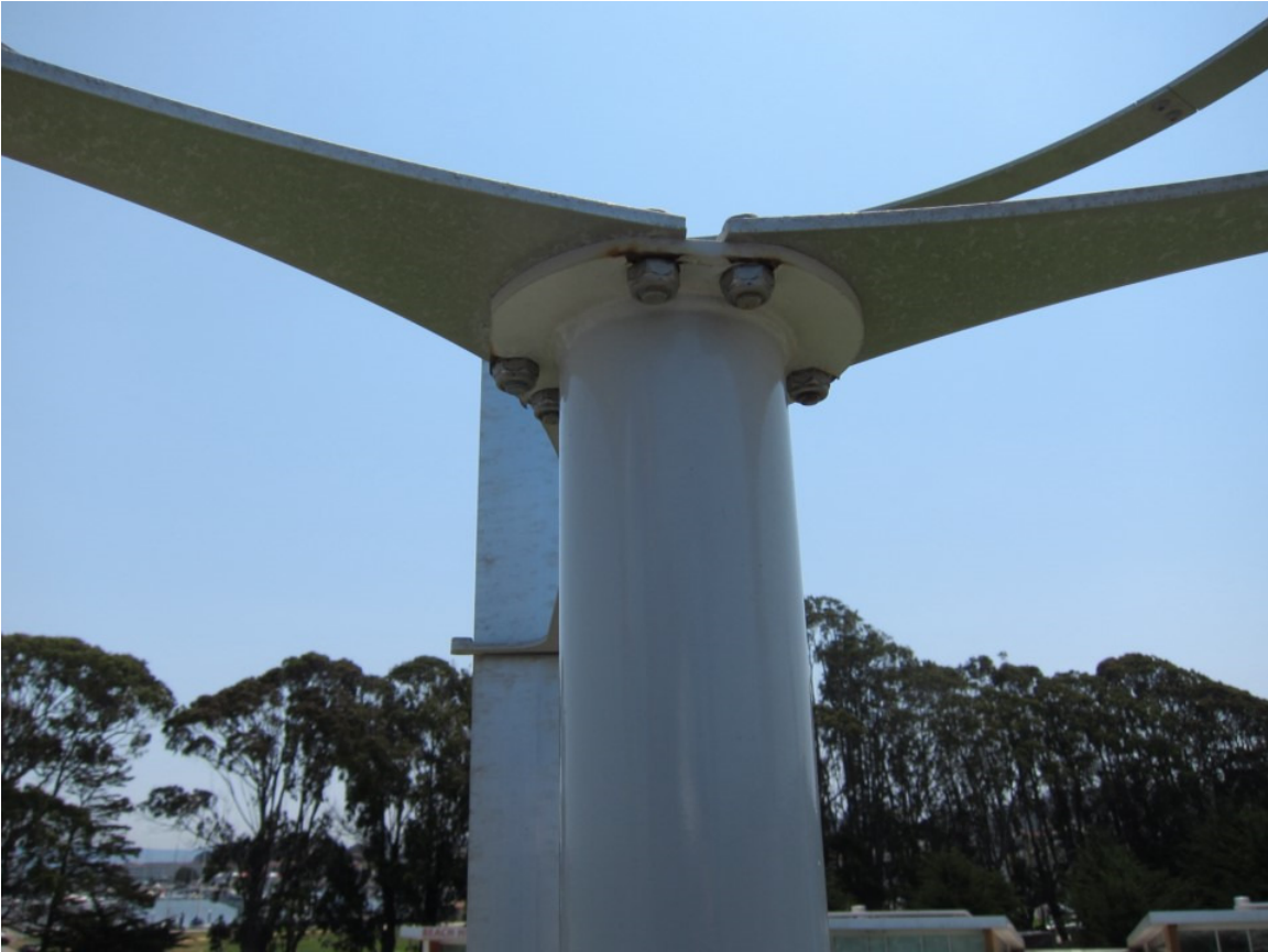
Figure 1. Northern Windspire. Rust is occurring at bolted flange connections on the rotor. Cold galvanizing compound was applied.
