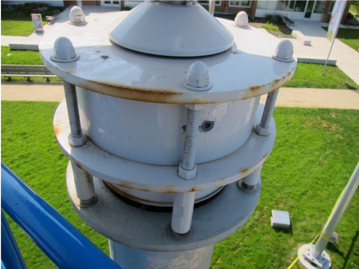
Figure 12. Generator housing rust.
