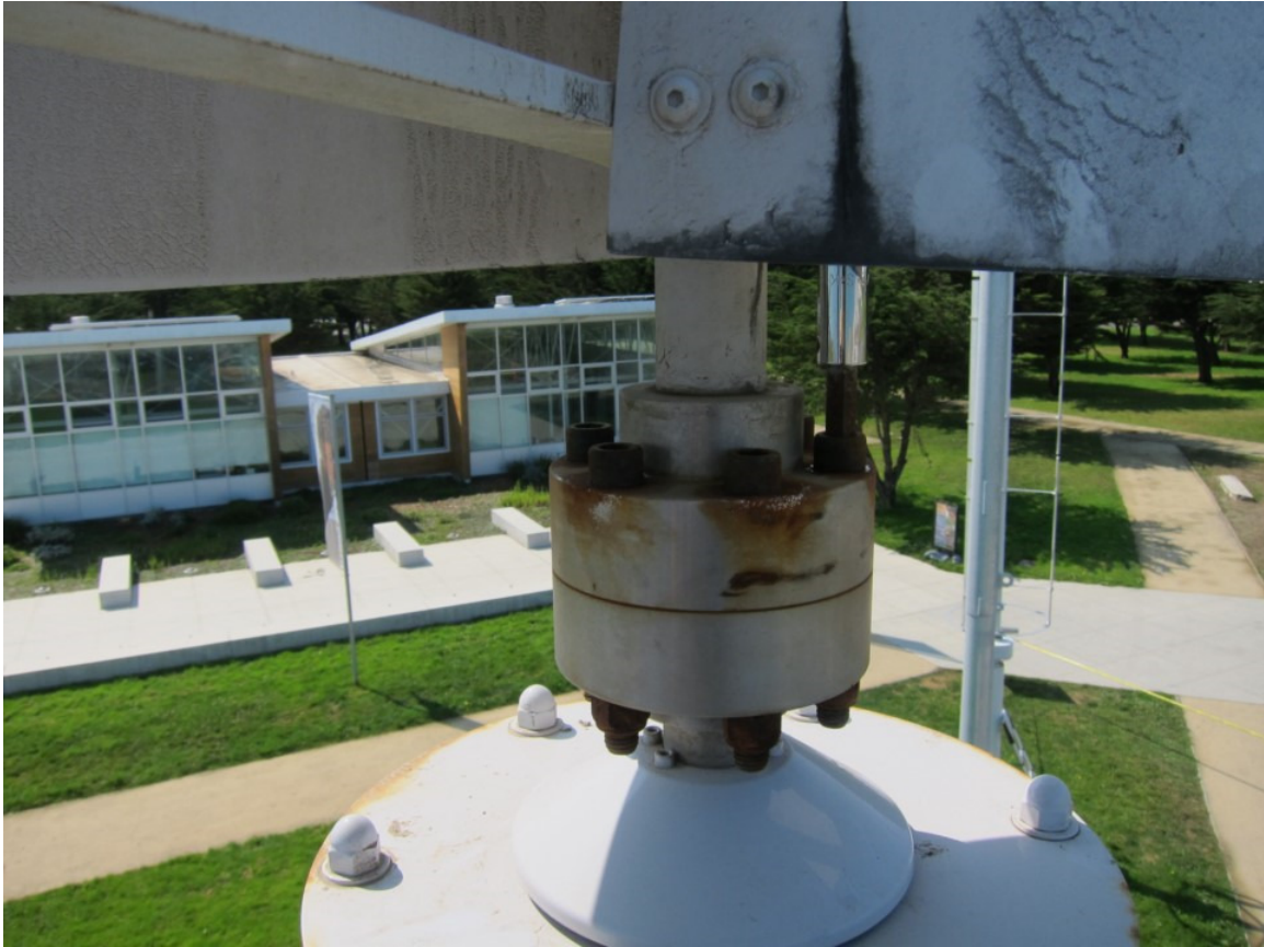
Figure 11. Tangarie. Shaft bolt rust.
