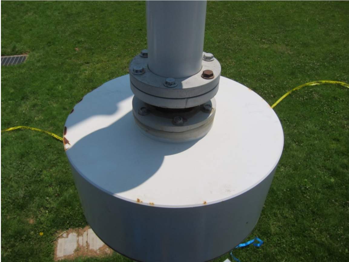
Figure 3. Northern Windspire. Rust present on inverter housing. Some cold galvanizing compound was applied but the rust will likely become worse.
