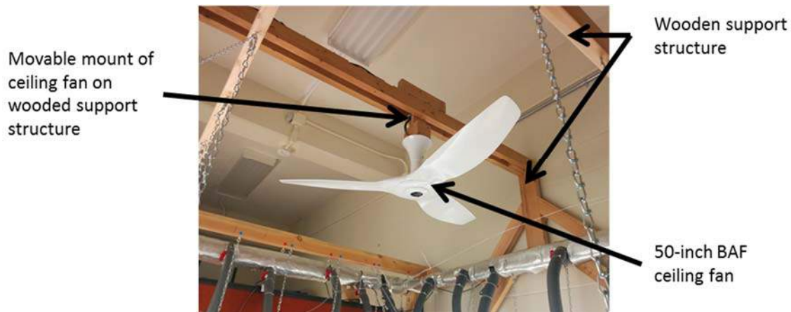
Figure 2.2.1: Ceiling fan installation
