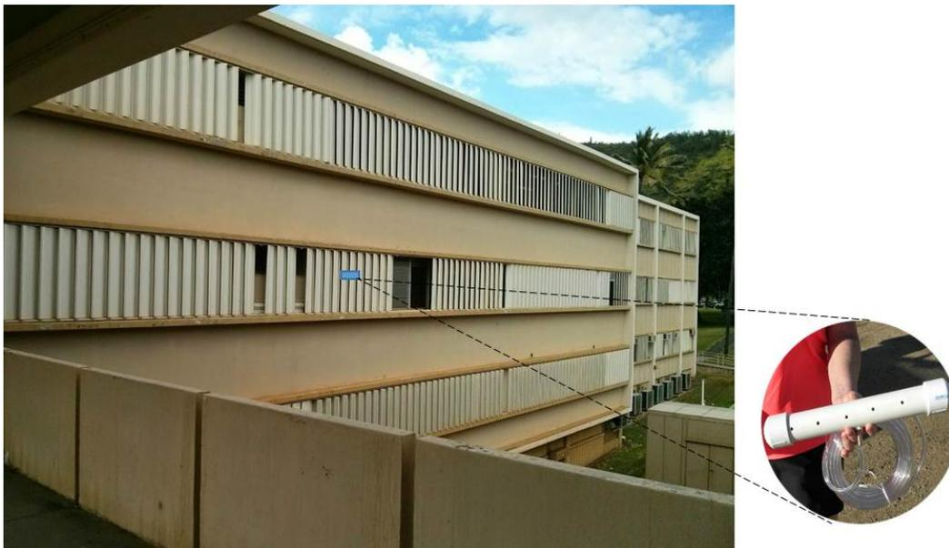
Figure 3.2.19: Location of four pressure tubing terminals installed on the South façade of Keller Hall – the terminals are installed behind the vertical shading panels
