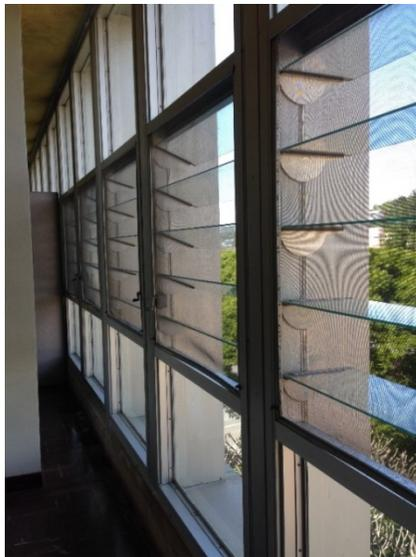
Figure 4.6: North wall of Sinclair room 301 with window panes and glass louvers.
