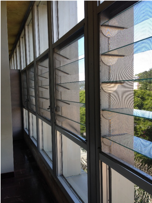
Figure 4. 5: North wall of Sinclair room 301 with window panes and glass louvers.
