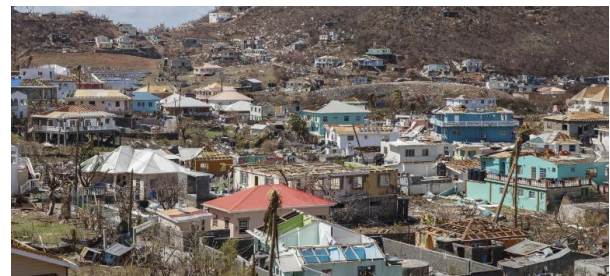
Figure 2. Homes destroyed by Hurricane Beryl in 2024.
