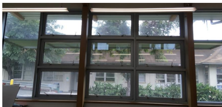
Figure 5. The bank of nine operable windows on the south side of the buildings. The three windows on the left side are wired with sensors to indicate if at least one window is open.
