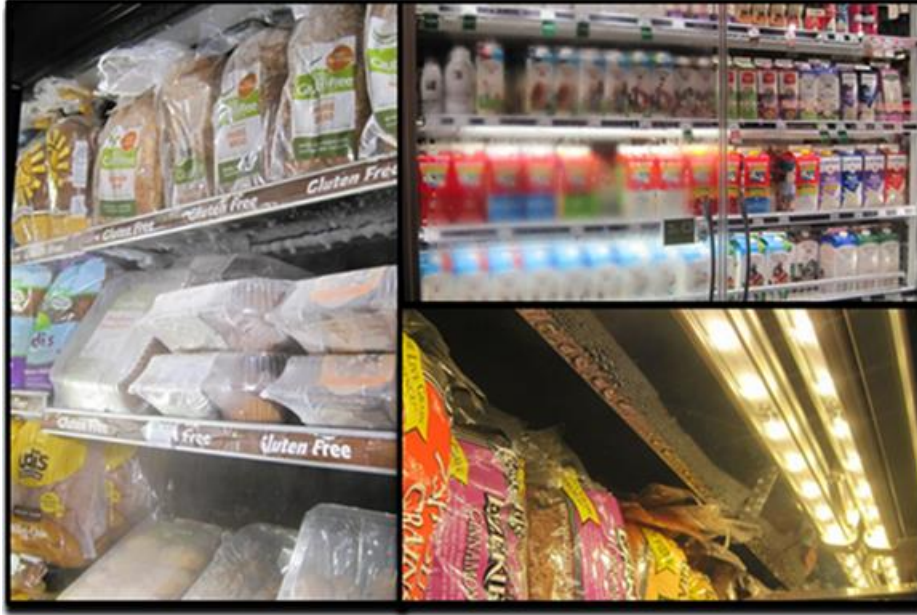
Figure 2–34 Effects of high humidity on grocery store refrigeration, Whole Foods, Kailua, Hawaii, summer 2013 (Credit: Ian Doebber/NREL)
