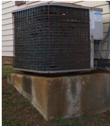
Photo 2. Compressor on concrete pad protects it.
