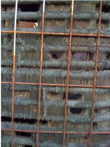
Photo 1. Corroded cooling fins.
