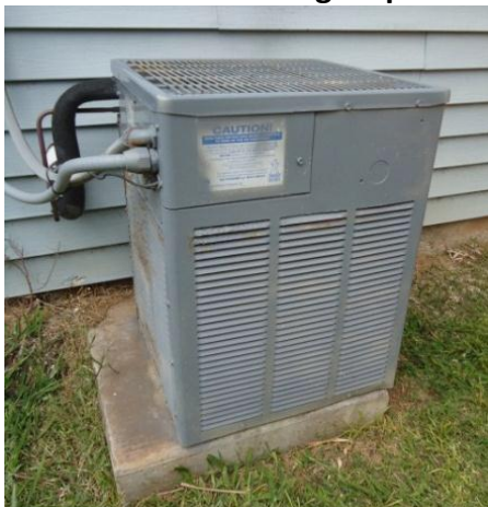
Photo 5. Good cooling fin protection.
