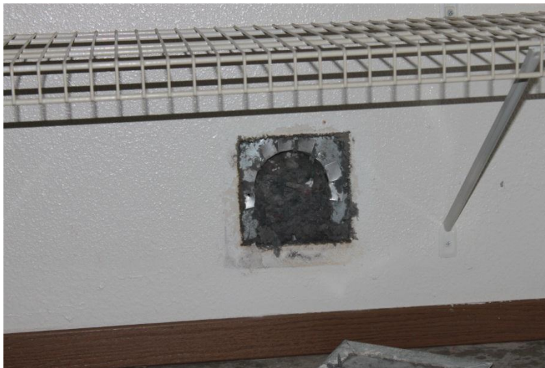
Photo 8. Clogged dryer duct in an empty home.
