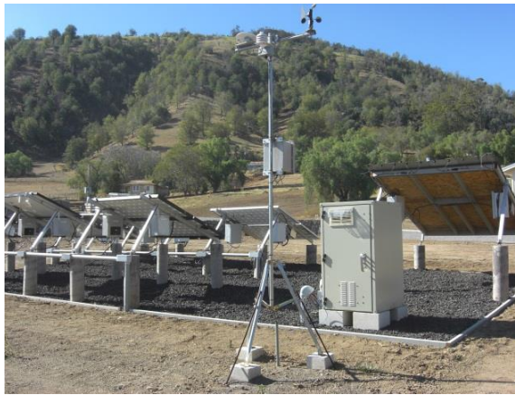
Figure 4.5 Weather Station/DAS Enclosure
