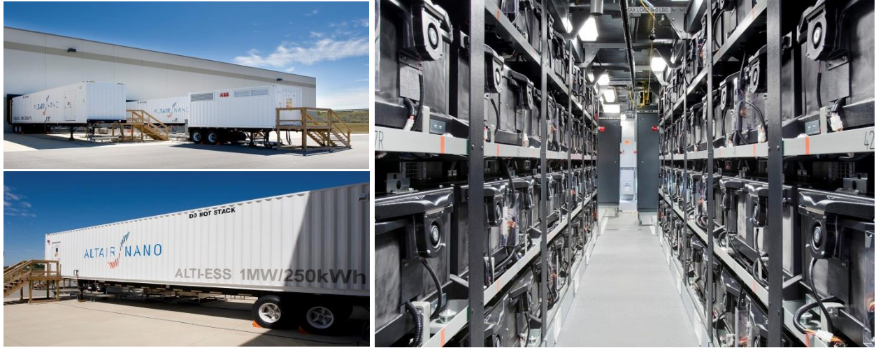
Figure 4.1 ALTI-ESS Battery System (photographs courtesy of Altairnano Technologies)
