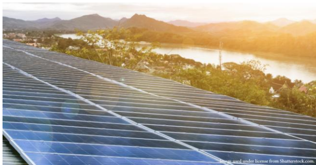
Figure 1. Rooftop solar PV array in Luang Prabang, Laos.
