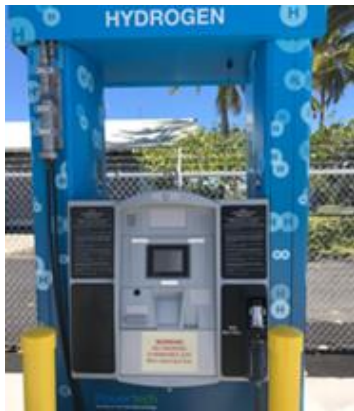
Figure 6. Hydrogen station dispenser.
