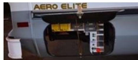
Figure 9. Bus export power unit.
