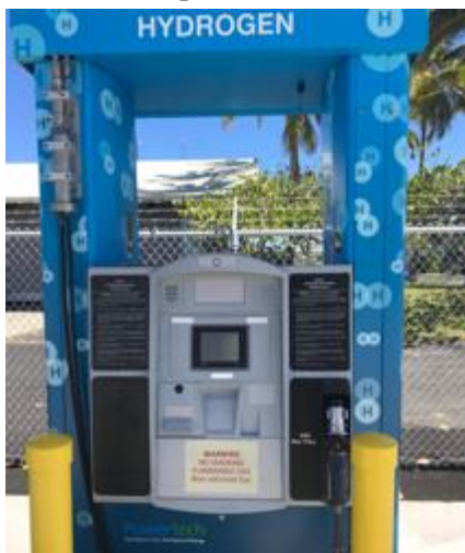
Figure 6. Hydrogen Dispenser.
