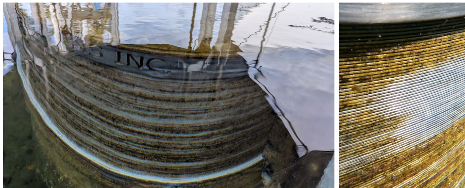
Figure 28. (top) Intake screen upon installation. (bottom) Intake screen after one year.
