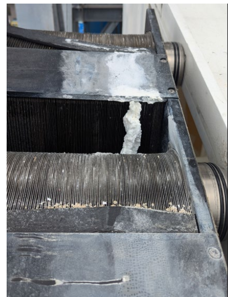
Figure 15. TFHX evaporator showing residue from ammonia leak and debris around the manifolds.
