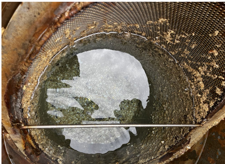
Figure 28. Strainer inspection revealed accumulated shells at the bottom and fibrous mats on the sides.
