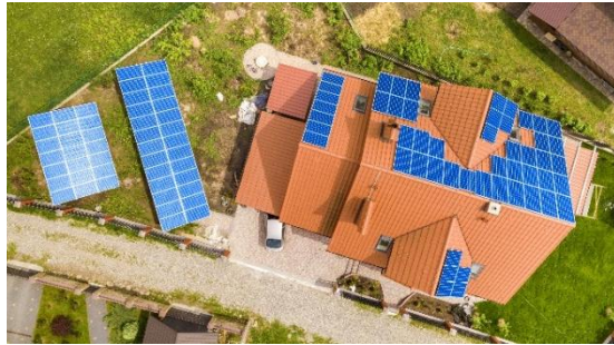
Figure 1. Rooftop solar PV system.
