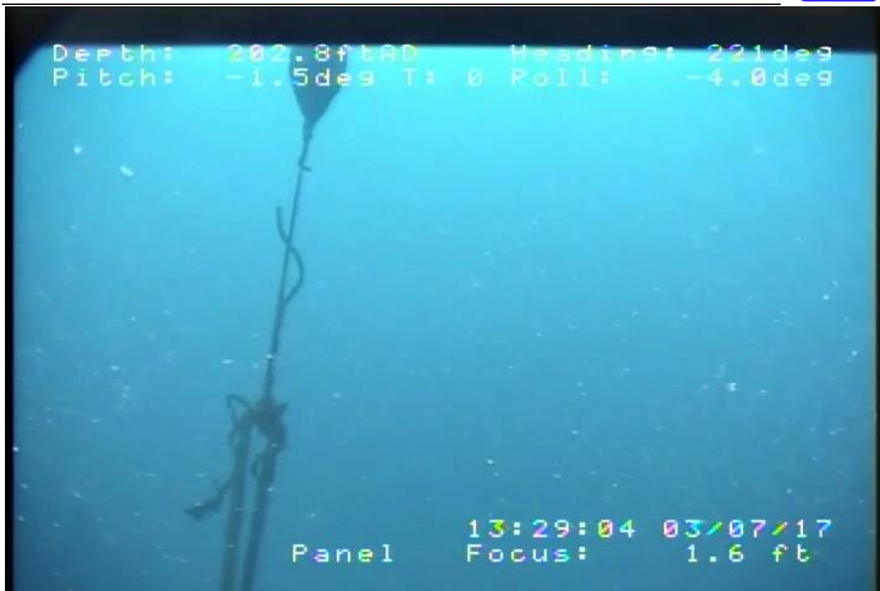
Figure 4-15 Line Loop near A2 Dip Section
