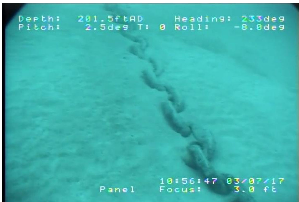
Figure 4-56 B3-ML-4 Kenter Link between SW5 and SW4
