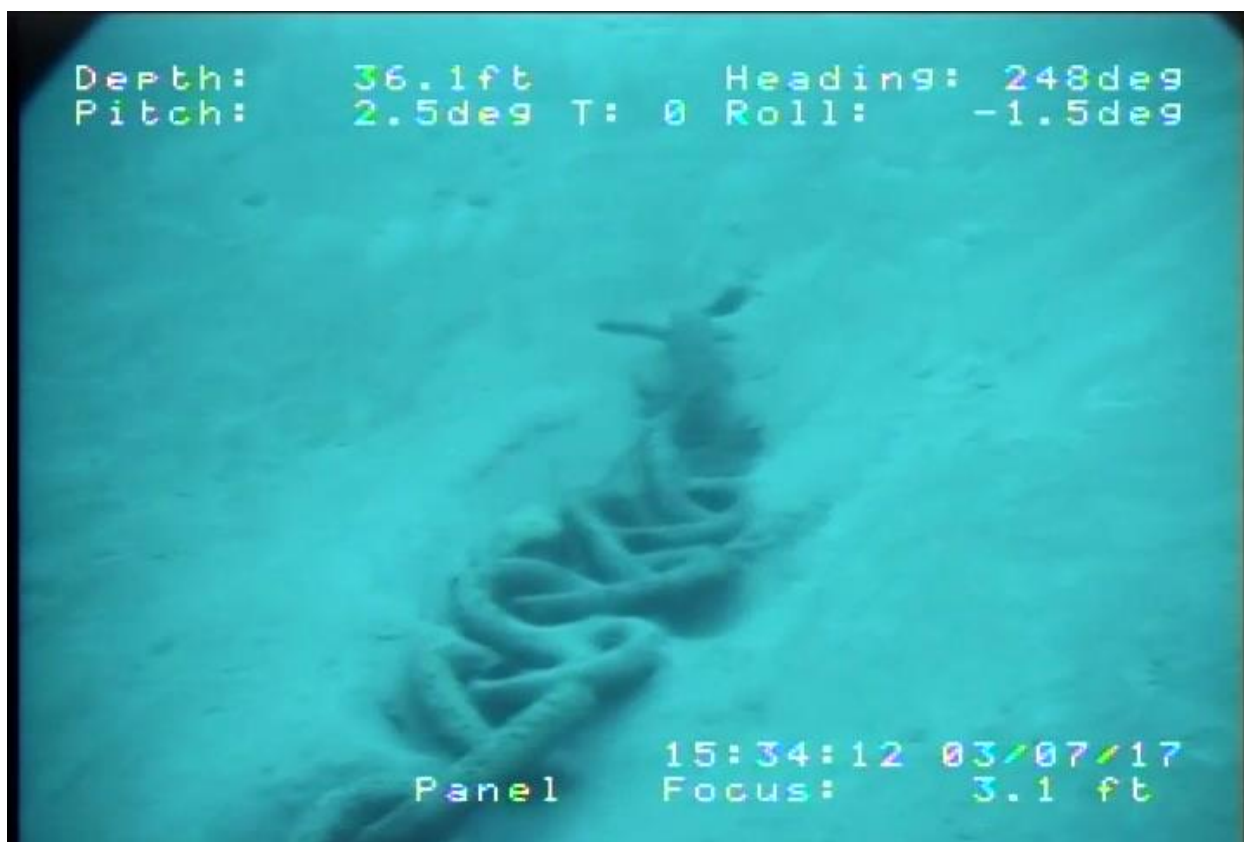
Figure 4-36 B1-ML-4 End of chain attached to anchor
