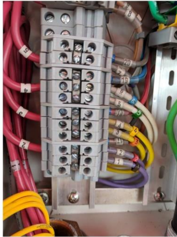
3-phase 440V with neutral connections for thruster power (3 wires for deck cable side)
