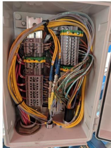
Fiber routing with all connectors.
