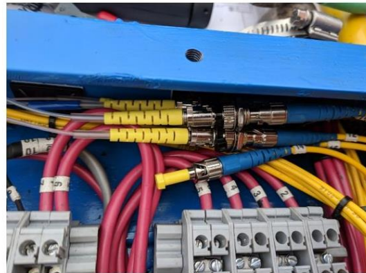
Fiber connections are tie wrapped to the wall of the junction box so to not move when rotating in the winch drum
