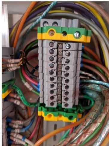
grounded in together in the fixed JB.
