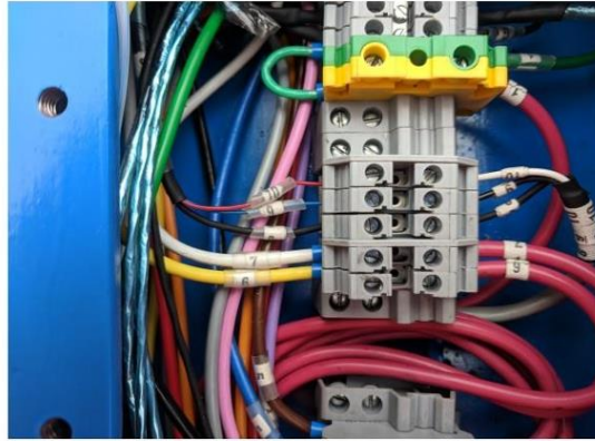
Single Phase 240V power (6,7) and CP probe twisted pair (8,9,10)
