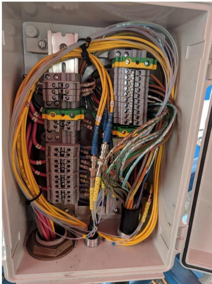
Figure 3-1. Fixed Junction Box Modification
