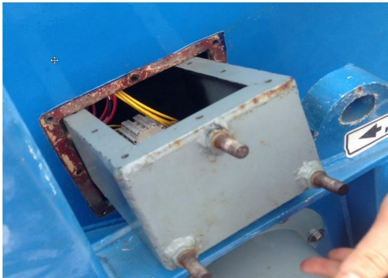
Old Rotating Junction Box, does not fit with the lid and hardware installed.
