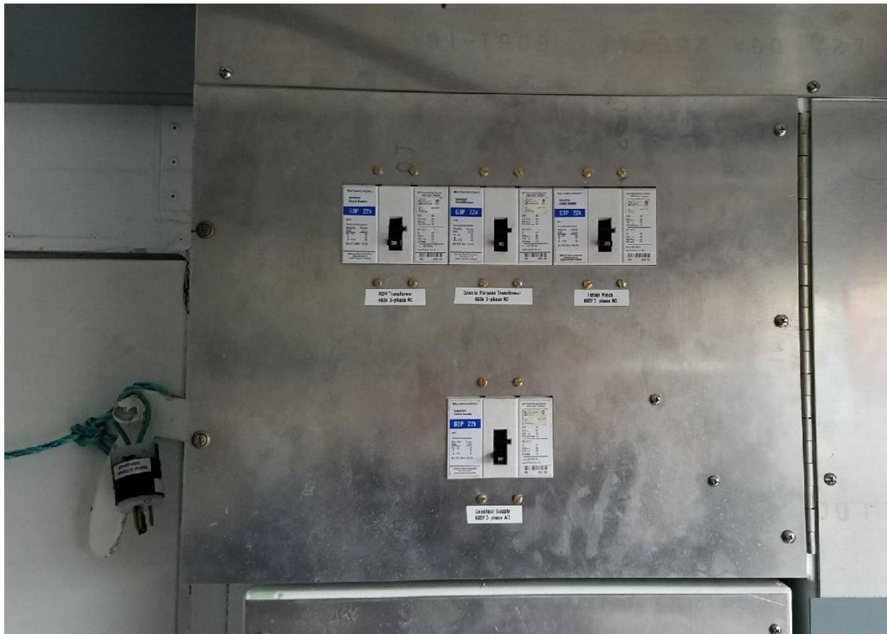
Figure 4. Power Distribution Panel
