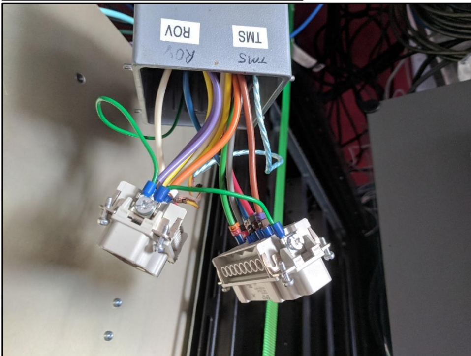
Completed connection wiring
